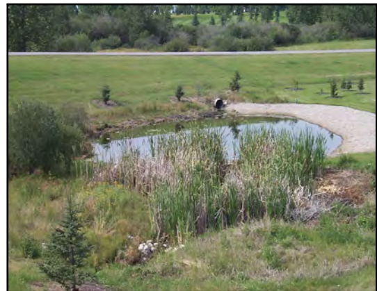
Stormwater pond in a residential community
