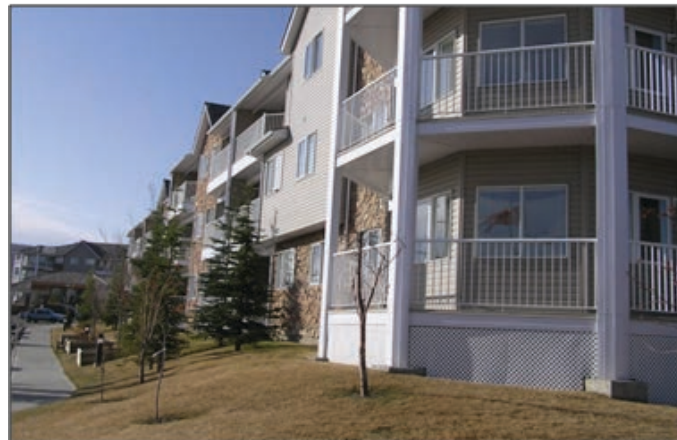
Figure D39: This photo shows a multi-unit residential structure with no entryways facing the street. The interface between building and street is not considered an acceptable design standard in an Activity Centre.
