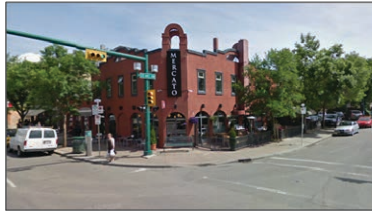
Figure D31: This image, a corner along 4th street S.W. in Mission, demonstrates ideal streetscape design for an Activity Centre. In this case, the building provides active fronts on both streets with parking accommodated on-street or in a small area behind the building.
