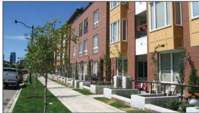
Figure D38: This multi-unit residential building, also in Bridgeland, has townhouses at grade, each with their own point of entry from the sidewalk. This demonstrates acceptable design in an Activity Centre.
